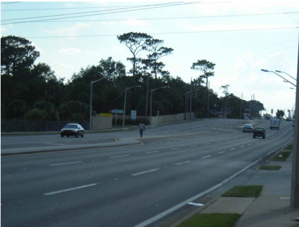
Figure 20 Silver Star Road at Belco Drive, looking west
