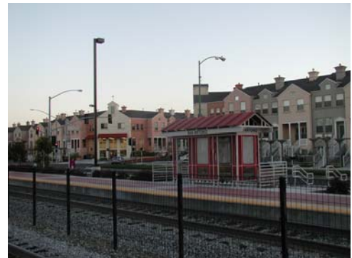
Apartments and retail served by a light rail station in Mountain View, CA.
